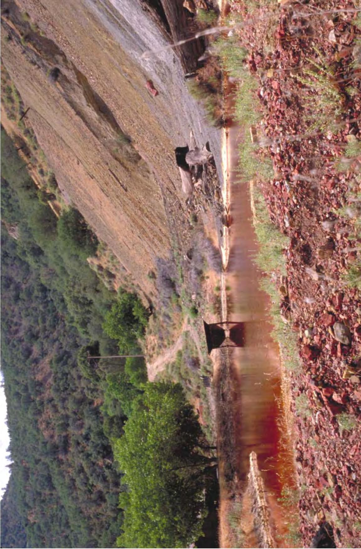
Figure 4: Piles of waste rock eroding into a non-functioning settling pond that discharges into San Carlos Creek.
