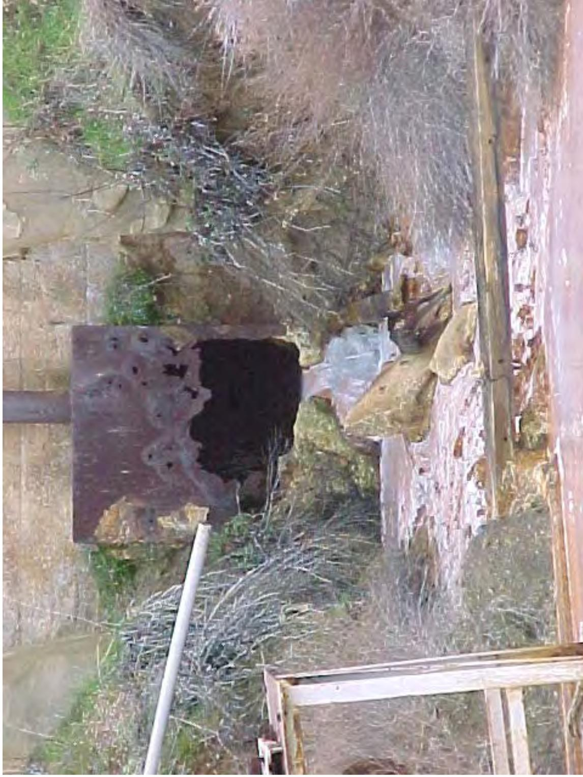
Figure 3: Discharge of acid mine drainage from the 10-level adit
